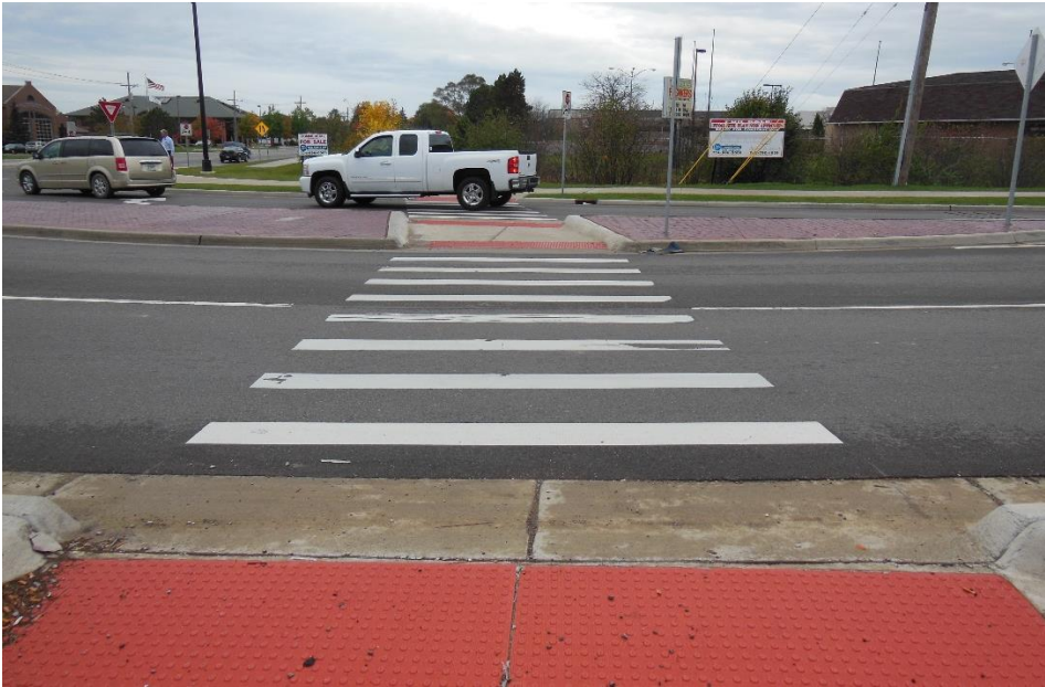
Figure 1. A crosswalk with a cut-through island with truncated dome DWS on the curb ramps and the island. [Source: J.M. Barlow]
